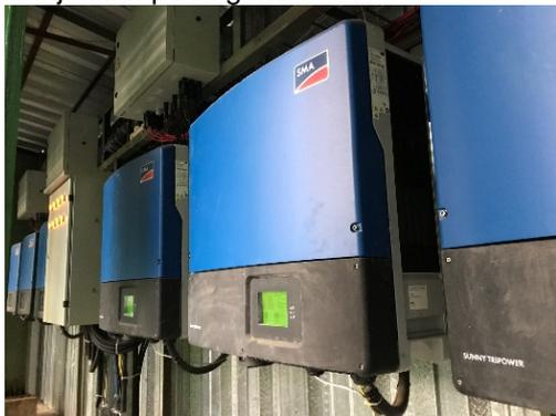
**Gambar 6. Inverter Sunny Tripower 20000TL [5]**
