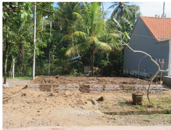
b. The foundation was being constructed be using concrete brick
