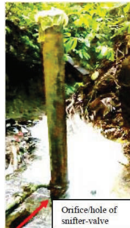
Figure 1. Orifice of the snifter-valve
