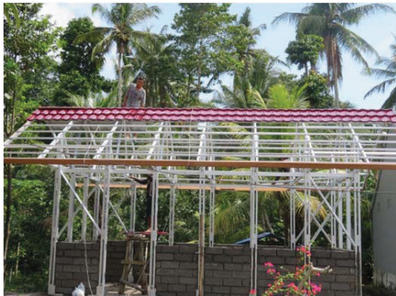
c. The structural system of light steel and brace were being constructed
