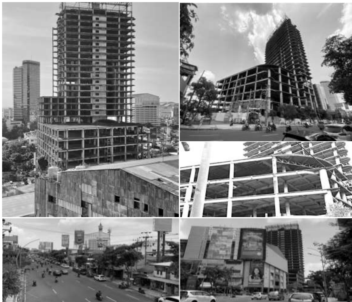
Figure 4. Situation Around the Abandoned Building.
