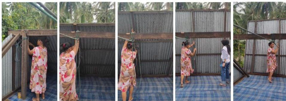
Figure 11. The process of opening the roof
