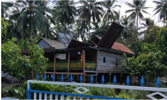
Figure 10. View of the roof when open
