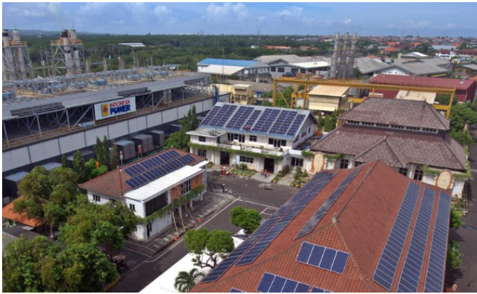
Gambar 14: PLTS on-grid Indonesia Power kapasitas 136 kWp [15]
