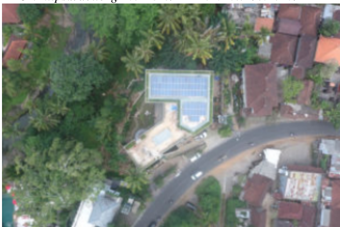
Gambar 10: PLTS on-grid Ubud Yoga Centre kapasitas 20,4 kWp [10]
