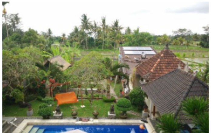
Gambar 8: Sistem PLTS on-grid Boogaart Residence kapasitas 2,4 kWp [10]
