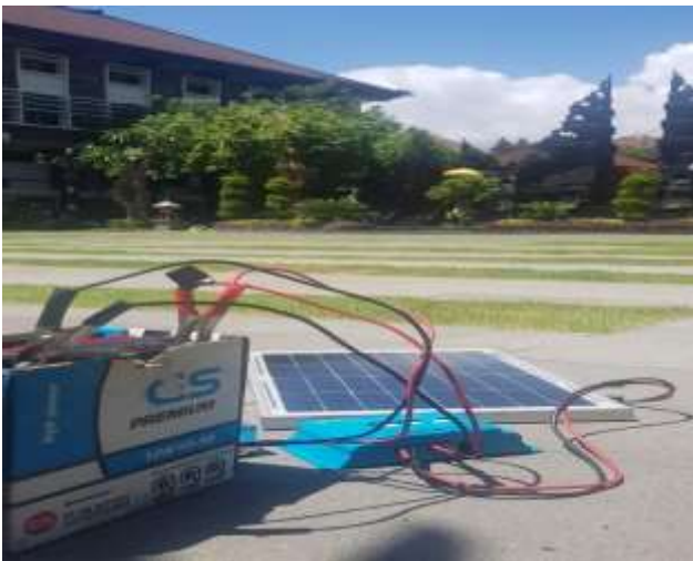
Gambar 7. Instalasi Solar Panel
