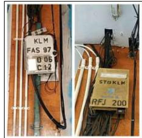
Gambar 6: ODP (*Optical Distribution Point*) Type Wall
