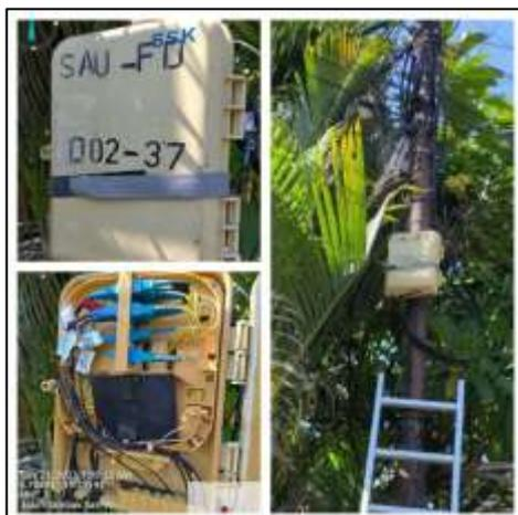
Gambar 8: ODP (*Optical Distribution Point*) *Type Pole*
