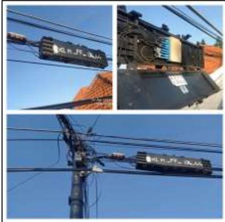
Gambar 7: ODP (Optical Distribution Point) Type Closure
