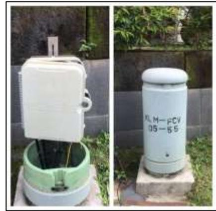
Gambar 5: ODP (*Optical Distribution Point*) Type Pedestal
