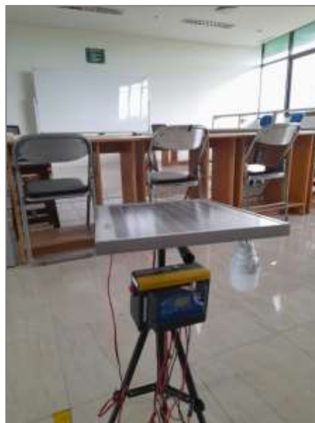
Figure 10: Testing Monitoring Solar Panel
