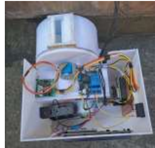
Figure 12 Installation of Electronic Devices
