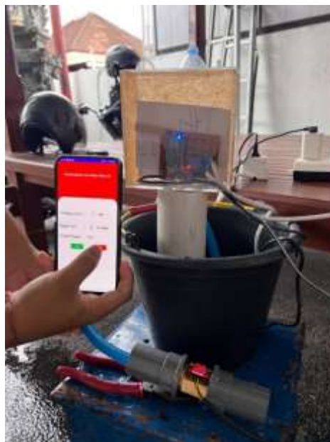
Figure 11 Test Turning Off the Relay
