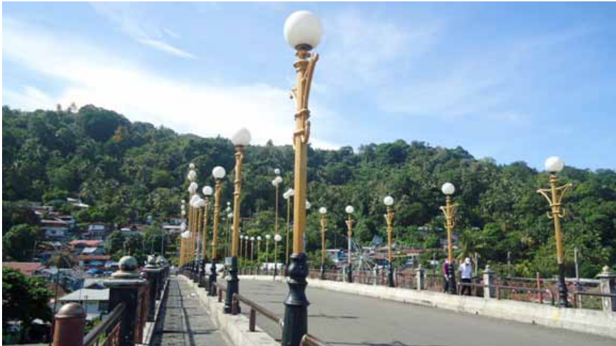
Photo 1. Siti Nurbaya Bridge in the days (Personal collection)
