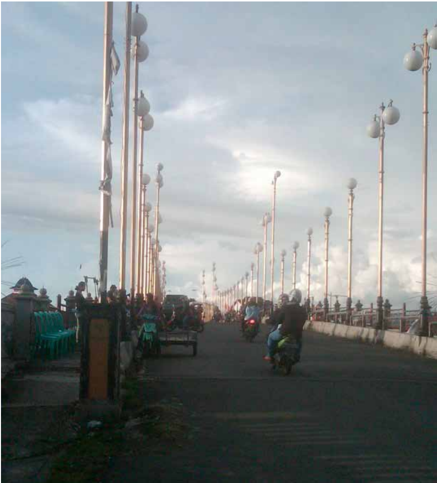
Photo 2. Siti Nurbaya Bridge in the days (Personal collection)
