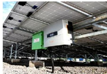
Gambar 8. Grid-connected inverter SUNGROW SG20KTL
