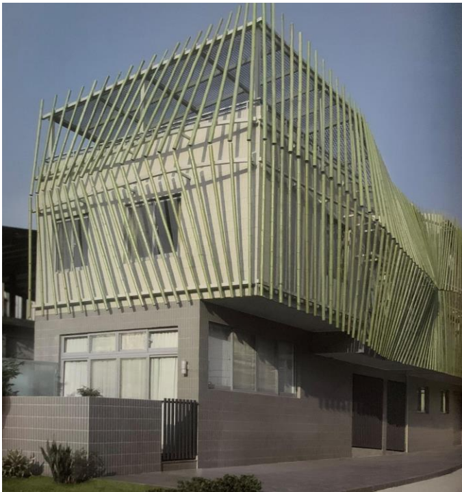
Fig. 7 Bamboo Forest House-ROEWU architecture-Luo-ong,Taiwan,2008 Literature:"Bamboo" by Àlex Sánchez Vidiella, 2011 Page 32 In this building the bamboo canes create the facade of the building.
