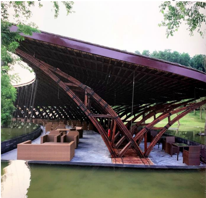
Fig. 8 Bamboo Wing-Vo Trong Nghia-Phúc Yên,Vietnam,2009 Literature:"Bamboo" by Àlex Sánchez Vidiella, 2011 Page 288 The construction after the completion of the building.
