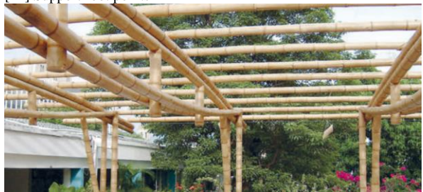
[15] Stacked beams and prestressing
