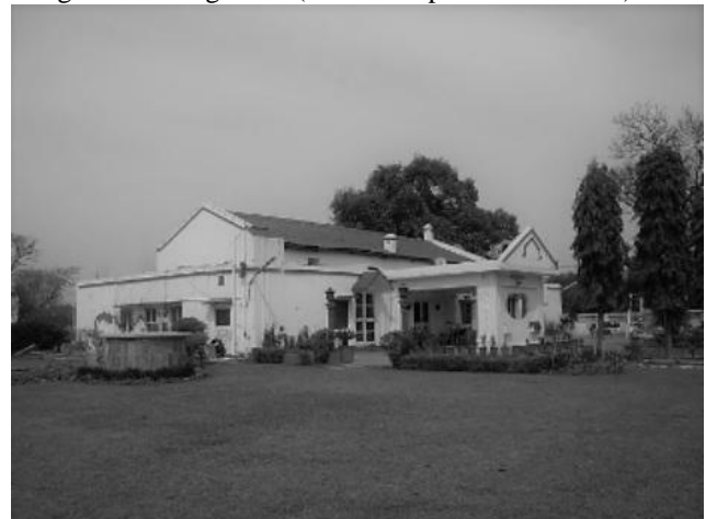
Figure 1. A Typical Bungalow in Ambala Cantonment area, standing in the middle of a huge plot.
