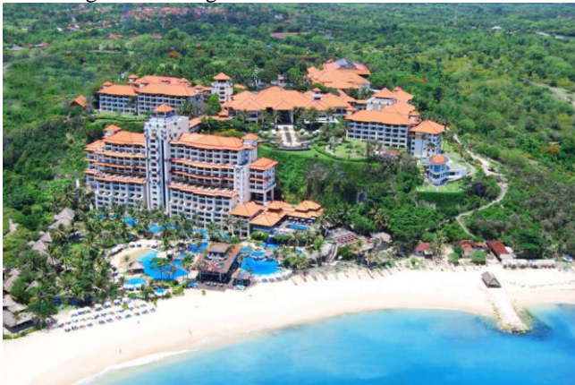
Figure 6. Bali Hilton Resort, Nusa Dua - Clearly pushing the limits of legal construction.
