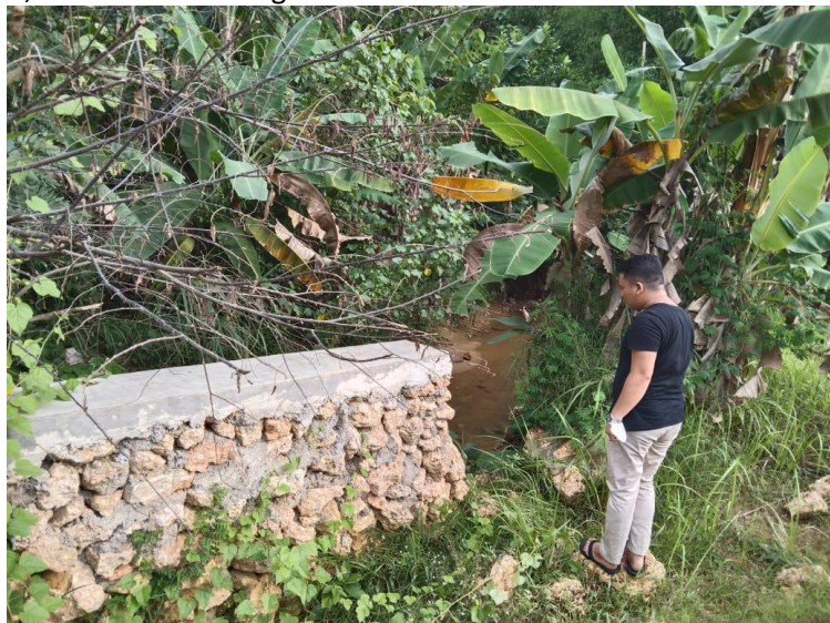
Figure 3: Construction of TPT
