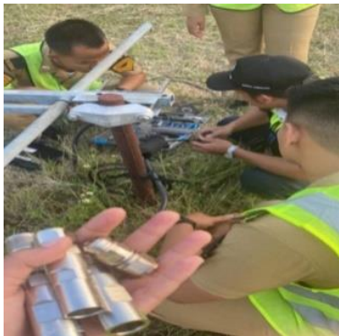
Fig. 9 Installation of N Type Male Connectors
