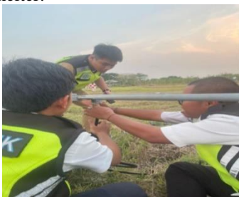
Fig. 10 Installation of Cable on Nearfield Antenna
