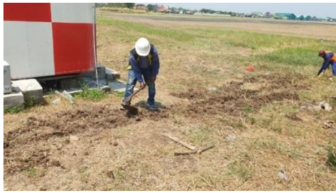
Fig. 8 Excavation and Cable Laying Work by Vendor
