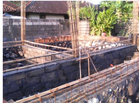
a. Foundation construction and bamboo reinforcement
