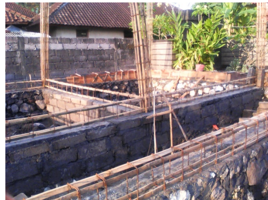
a. Foundation construction and bamboo reinforcement
