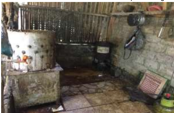
Figure 1. Construction of Chicken Slaughterhouses in Jampang Village
