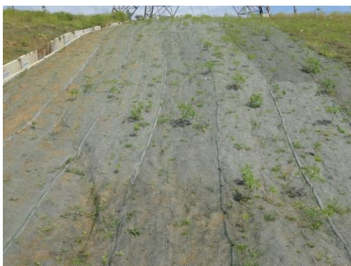
Figure 10. Whole view from the front after 3 months
