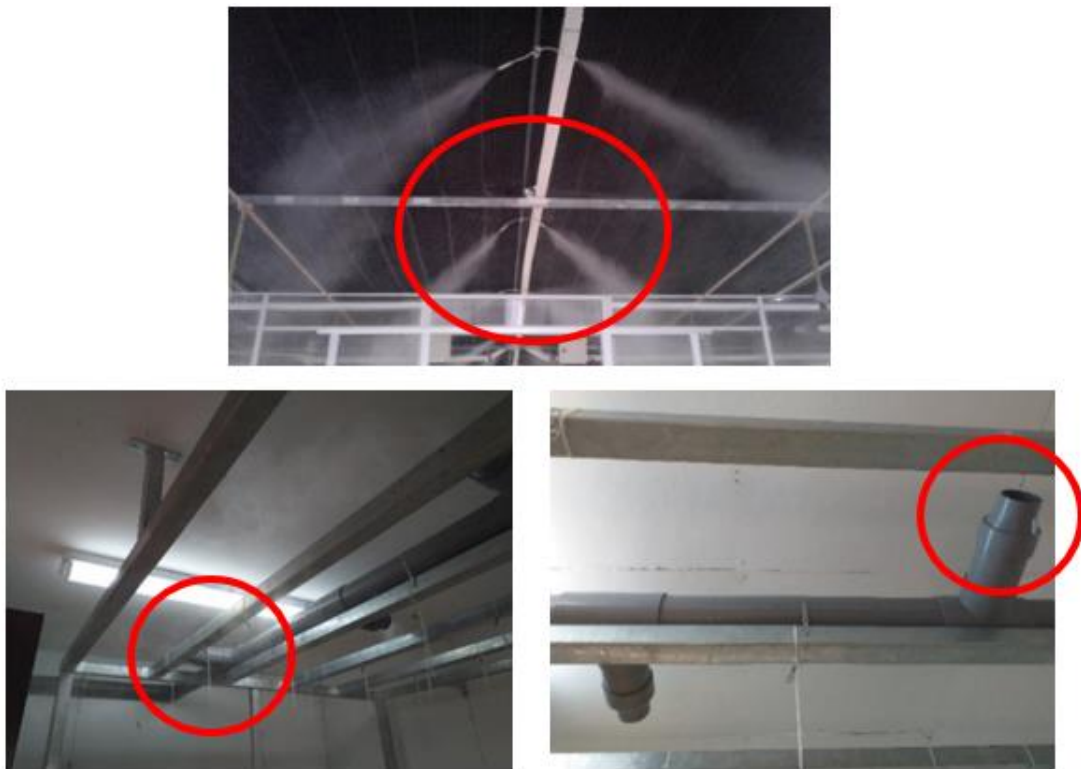
Figure 8. Water Sprinkle (top) and Water Vapor Spray (bottom) in a Mushroom House.
