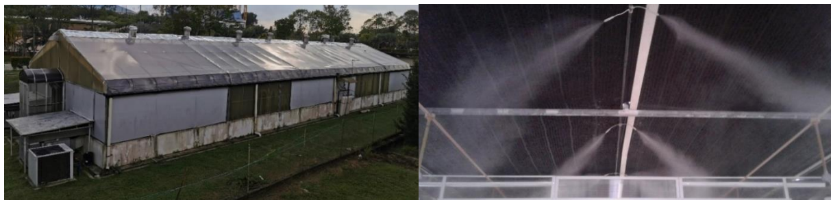
Figure 2. Control Environmental Mushroom House (CEMH) (left) and Control of Temperature and Relative Humidity by Automatic Water Sprinkle (right)
