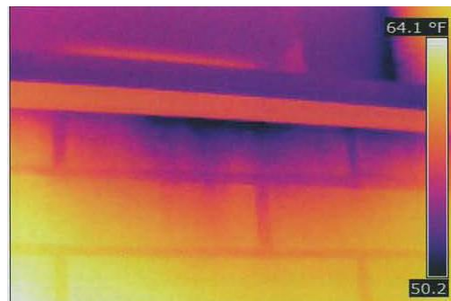
Fig. 2. Cool air infiltration through opening under window assembly.
