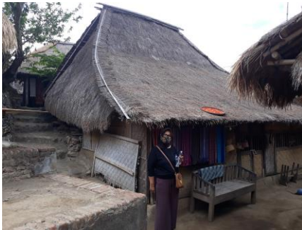
Figure 5. Building materials: alang-alang/thatched roof and bamboo walls
