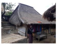
Figure 5. Building materials: alang-alang/thatched roof and bamboo walls
