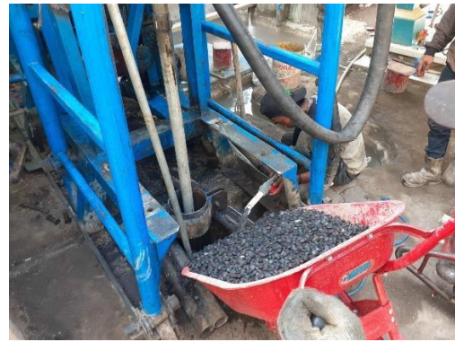
Figure 4. Charging Gravel Pack
