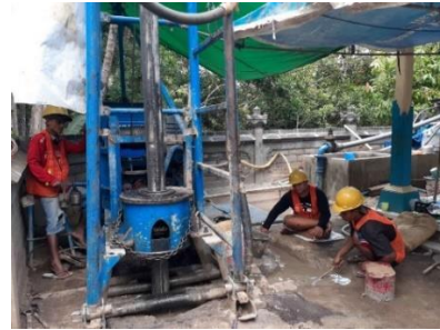
Figure 2. Drilling of groundwater wells (Source: BWS Bali- Penida 2019)
