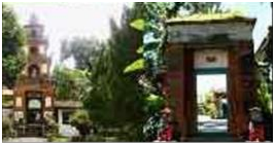
Fig. 4 Nista Mandala section functioned as a place for guests to prepare to enter the deeper castle area
