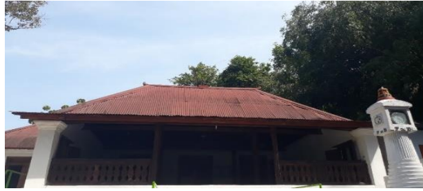
Figure 4. The Roof of Pajimatan Imogiri Mosque Source: Personal Documentation, 2019
