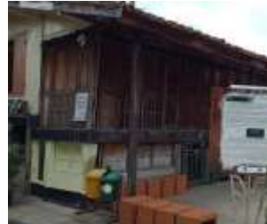
Limas House After Restoration
