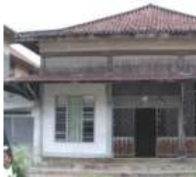
Stone House Before Restoration
