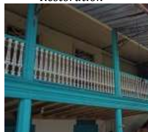
Sea Twin House After Restoration
