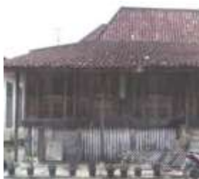
Limas House Before Restoration
