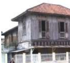
Land Twin House Before Restoration
