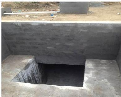
**Gambar 3a.** Sistem feeding (manhole)
